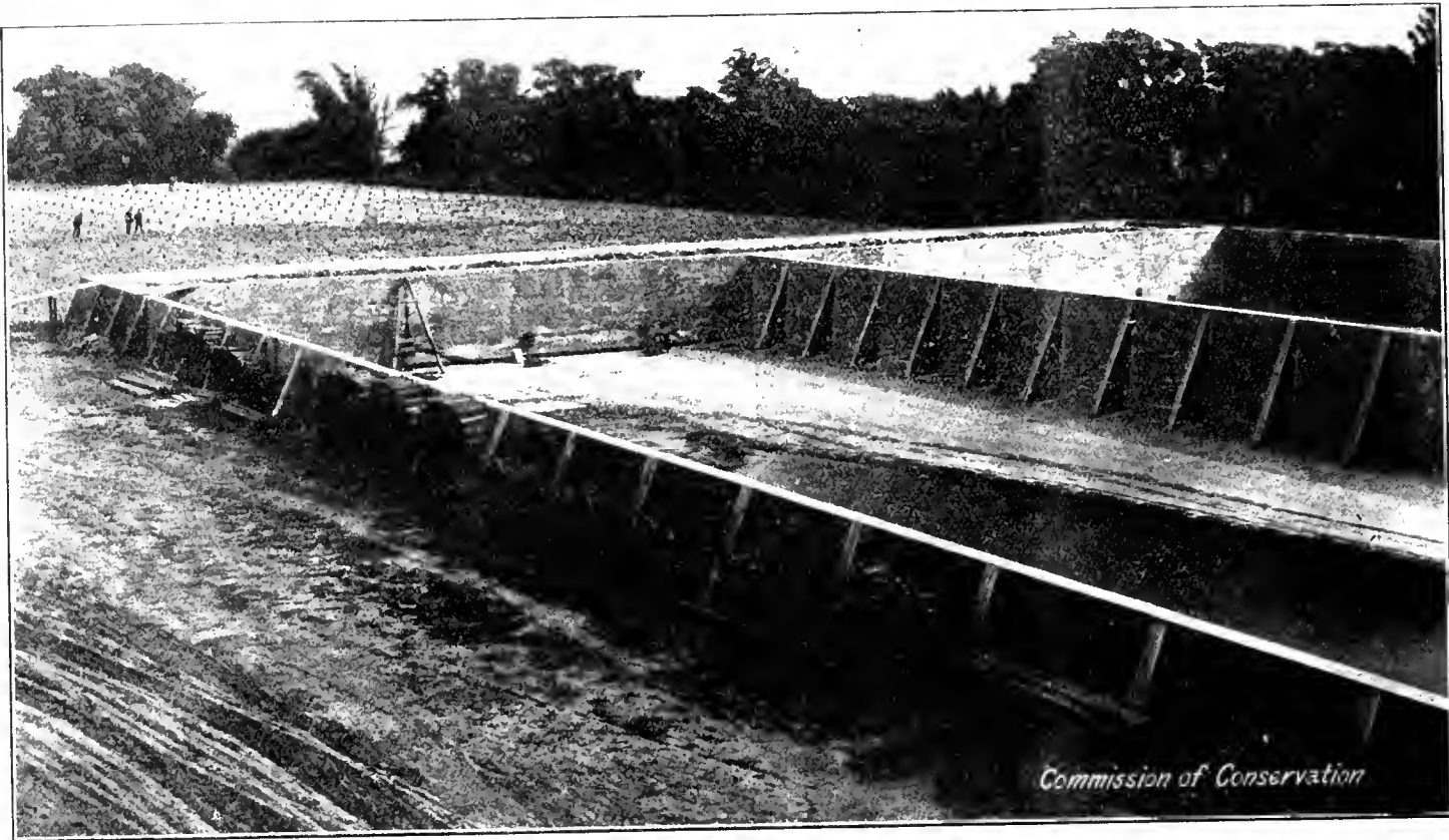
Hamilton Sewage Disposal Works—Tanks and Filtering Beds.
